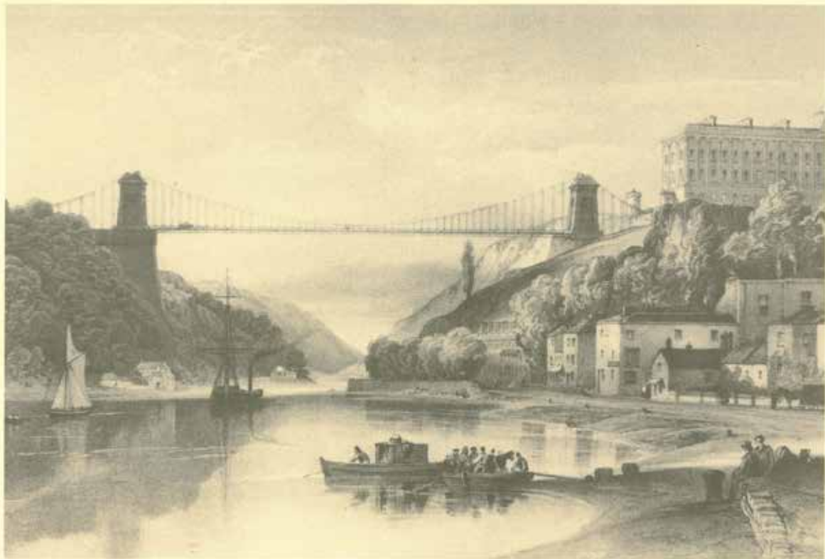
THE CLIFTON SUSPENSION BRIDGE, BRISTOL
